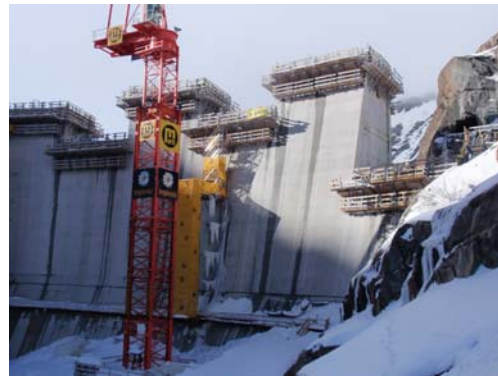
Fig. 2. Vieux Emosson Arch dam under construction (Schleiss 2013)
