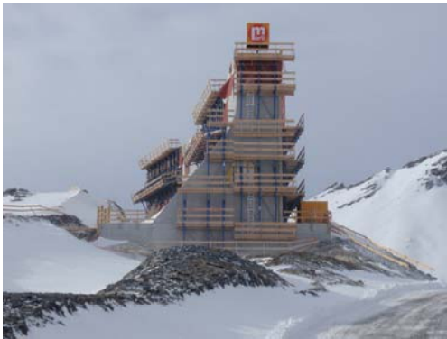
Fig. 1. Muttsee Gravity dam under construction (Schleiss 2012)
