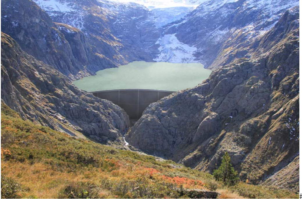
Fig. 3. Photomontage of the future 180 m high Trift dam, which uses the already freed valley by glacier retreat. #
