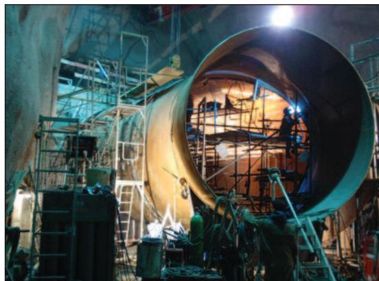
(a) Welding of a steel liner heading towards the underground powerhouse before backfilling with concrete (courtesy of A.J. Schleiss).
