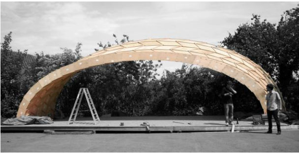
Figure 2: Double-layered timber plate vault prototype of the Multipurpose Hall Project (Annen SA, Manternach), scale 1:2 (12.5m span)
