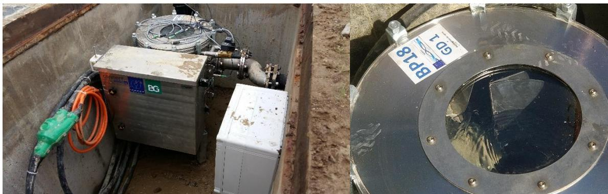
Figure 2: Installed prototype sealed vortex siphon (courtesy of BG)
